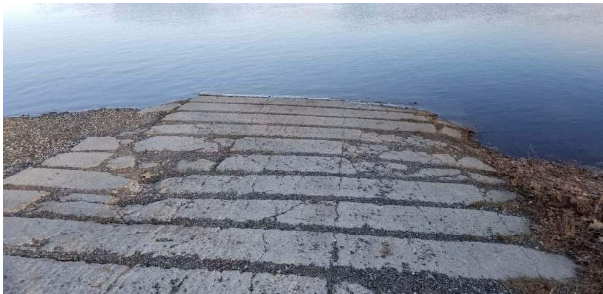
Photo 2 – Chelmsford Boat Access Ramp
