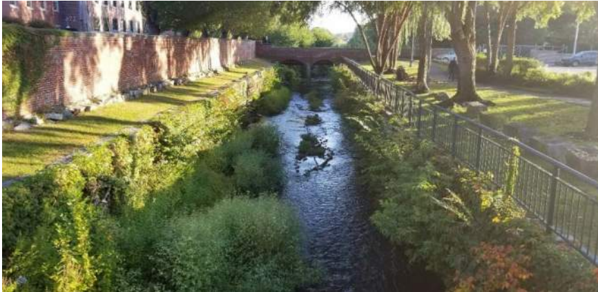
Polygon No.: 45 and 46 Photo No.: 45 Date: 9/26/2019 Direction Photo Taken: Northeastly Description: Vegetation growing on the eastern side of the canal wall (left side of the photograph) includes several tree species (i.e. mulberry, buckthorn, tree of heaven, etc.) and dense vines, including Boston Ivy and poison ivy. Vegetation growing on the western side of the canal wall (right side of the photograph) includes less trees than the eastern side of the canal and similar vine species.
