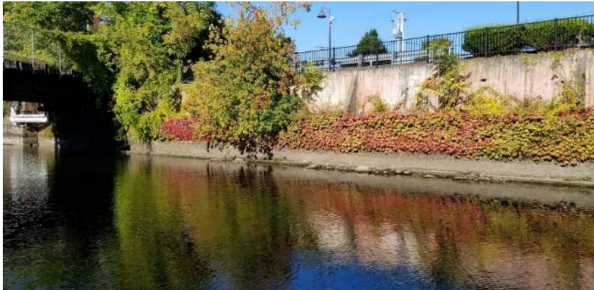
Polygon No.: 56 Photo No.: 56 Date: 9/26/2019 Direction Photo Taken: Southwesterly Description: Most of the canal wall is made of concrete with riprap placed at the toe of the wall. The vegetation growing on the canal wall consists of tree of heaven, box elder, and vines, such as Boston ivy.
