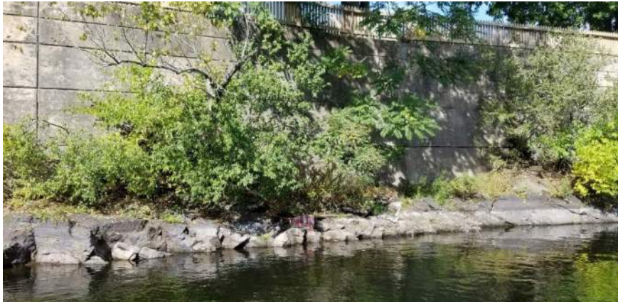
Polygon No.: 70 Photo No.: 70 Date: 9/26/2019 Direction Photo Taken: Northwesterly Description: The canal wall is primarily concrete with trees, such as locust and elm, growing at the toe of the wall.
