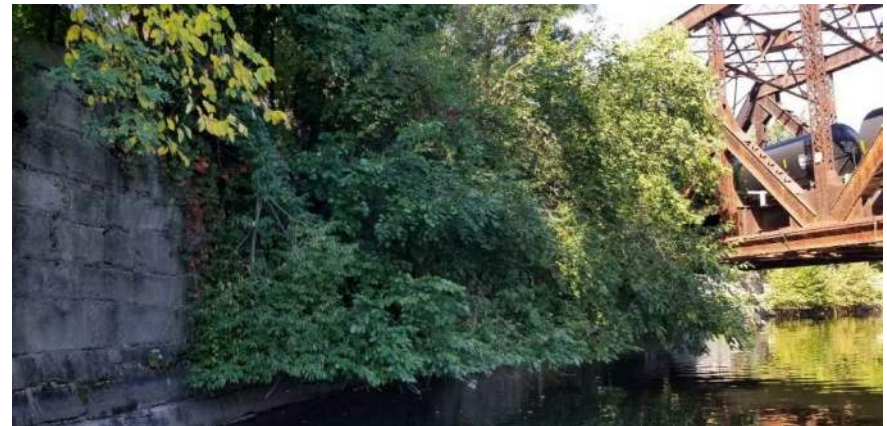
Polygon No.: 67 Photo No.: 67 Date: 9/26/2019 Direction Photo Taken: Northwesterly Description: Large locust and birch trees are growing on top of the canal wall.
