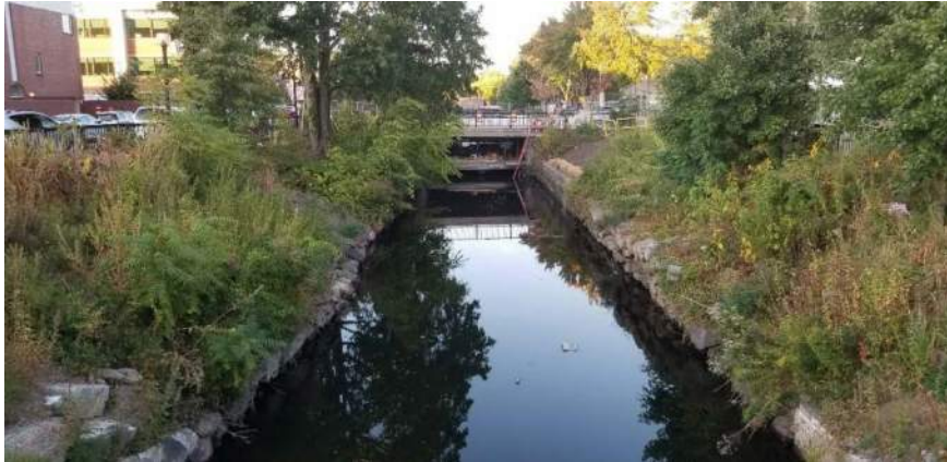
Polygon No.: 34, 35, and 36 Photo No.: 34 Date: 9/25/2019 Direction Photo Taken: Northeasterly Description: The vegetation growing out of the eastern side of the canal wall (right side of the photograph) is sparse and consists primarily of vines. The vegetation growing on top of and approximately 3 feet back from the western side of the canal wall (left side of the photograph) is primarily herbaceous.
