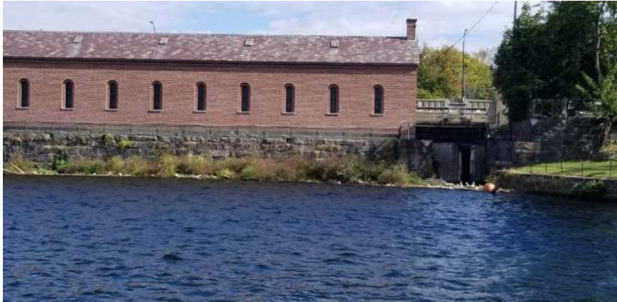
Photo Location No.: P-6 Date: 9/26/2019 Direction Photo Taken: Easterly Description: View of Pawtucket Gatehouse. Vegetation is growing on debris deposited against the gatehouse.
