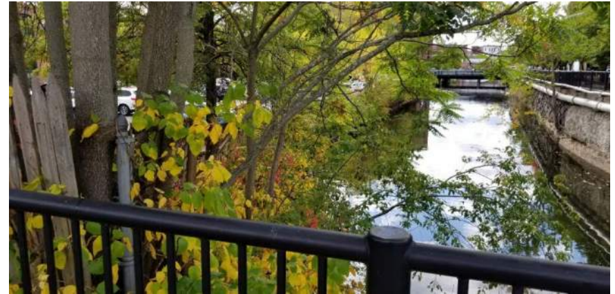
Polygon No.: 89 Photo No.: CV_Poly9 Date: 9/25/2019 Direction Photo Taken: Southeasterly Description: The vegetation growing out of the canal wall includes an approximately 10-trunked tree of heaven tree at approximately 6 inches diameter at breast height and poison ivy.
