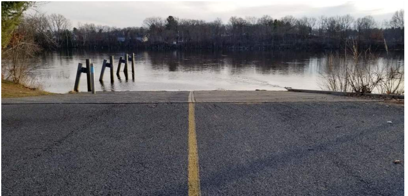
Photo 22 – Paved Rourke Brothers Boat Ramp
