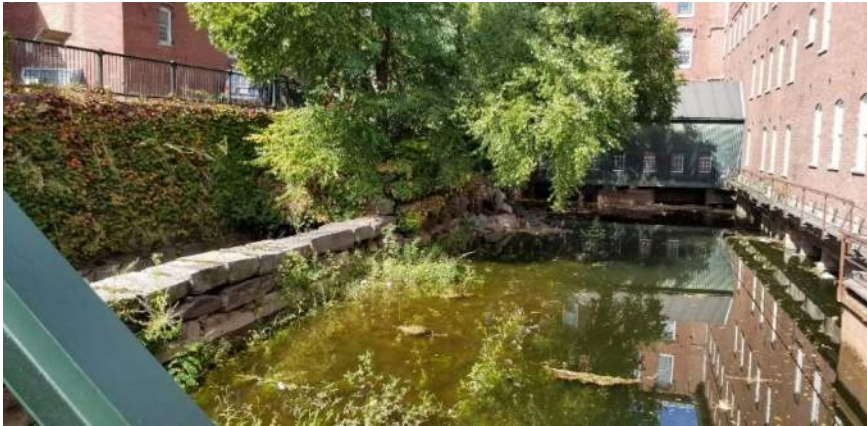
Polygon No.: 1 Photo No.: 1 Date: 9/25/2019 Direction Photo Taken: Northwesterly Description: Several large woody trees are located at the northwestern end of the canal, including river birch growing on top of the canal wall. Herbaceous plants including ragweed and Boston ivy dominate the western side of the canal wall (left side of the photograph).
